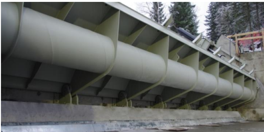
Photo 8 – Vanne clapet – Structure PRS mécanosoudée
